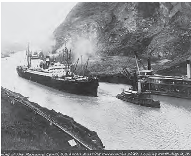
Shipping of the Panama Canal, S.S. Ancon passing Cucaracha slide. Looking north, Aug. 15, 1914
